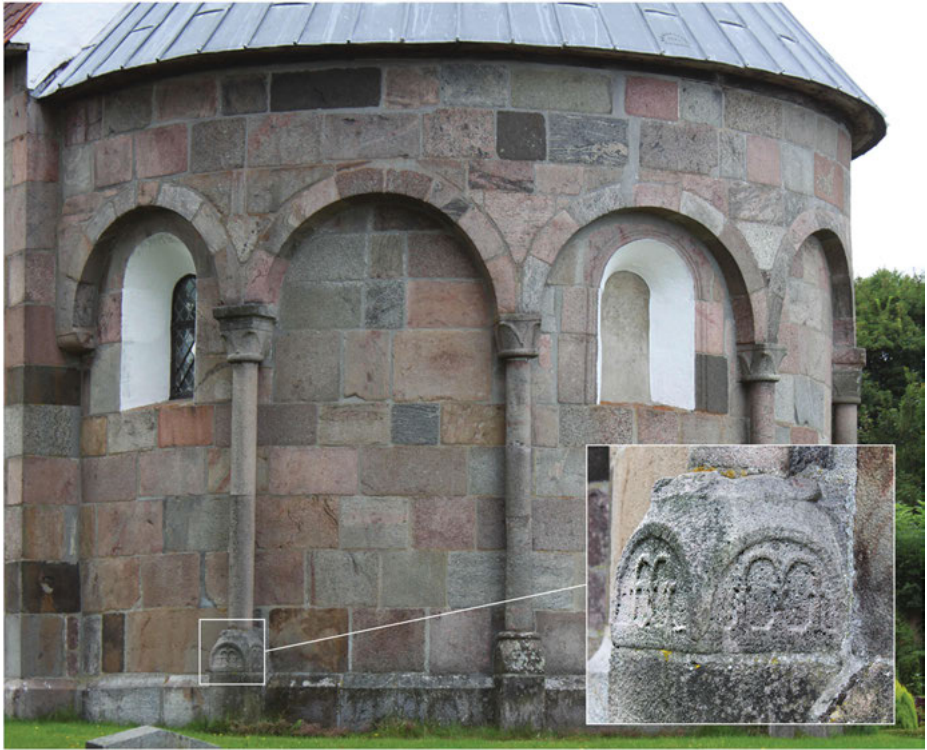
Fig. 15.6: Grønabæk Church, Central Jutland. a. Blind arcades, apse, exterior; b. Detail of column base from the blind arcade of the apse.
