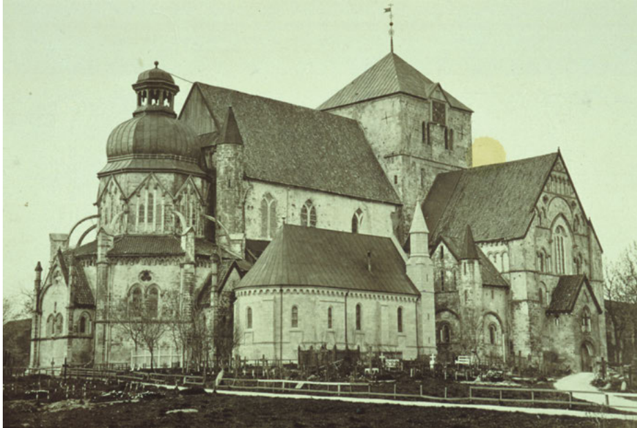
Fig. 14.2: Nidaros Cathedral, seen from the NE in 1872. The chapter house is restored, and the restoration of the octagon (to the left) is yet to begin. The Baroque cupola with its open lantern was soon after replaced by the present pointed spire, which is a reconstruction of the medieval roof.
