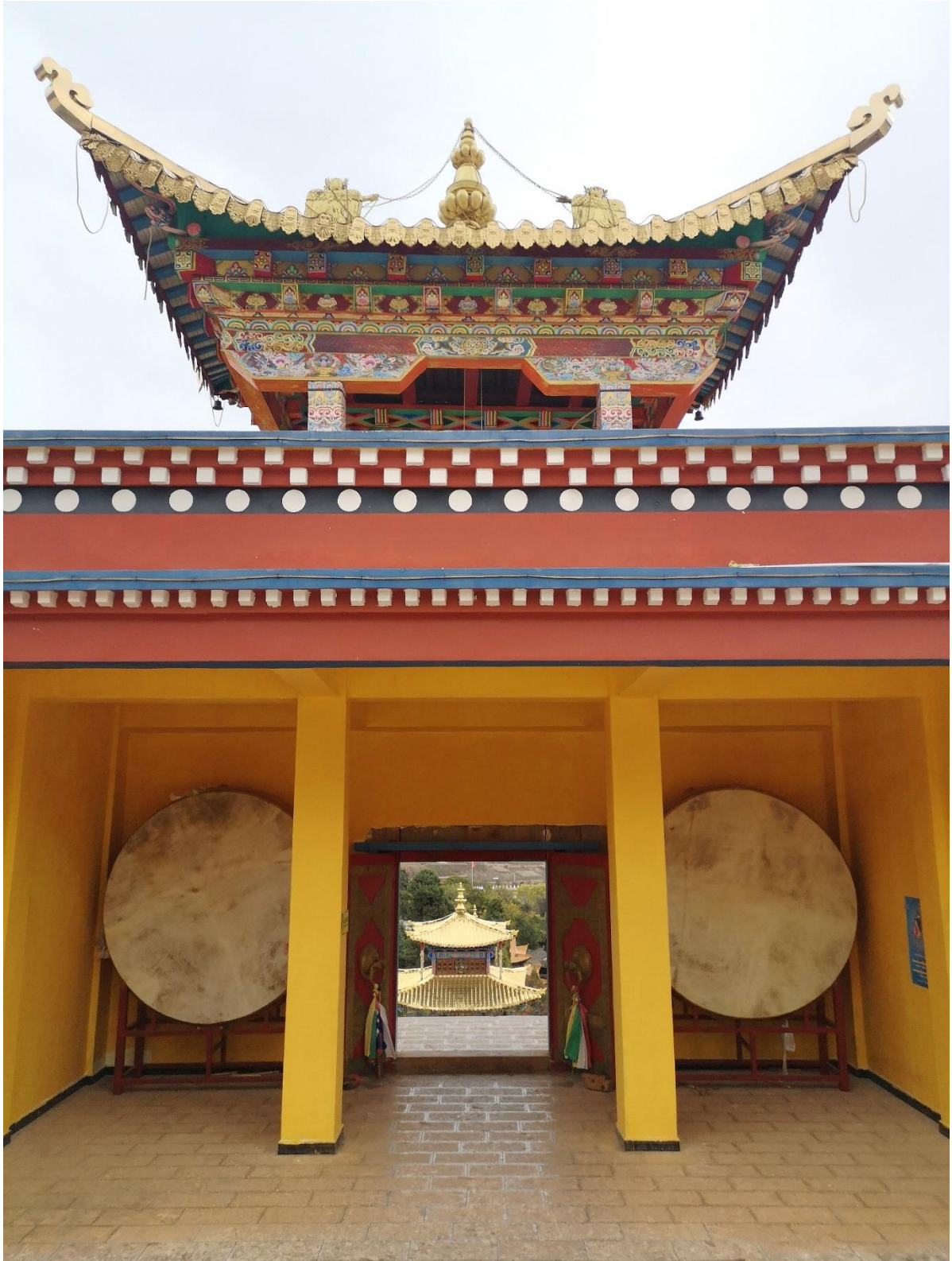
Figure 2 Entrance to the new addition.
