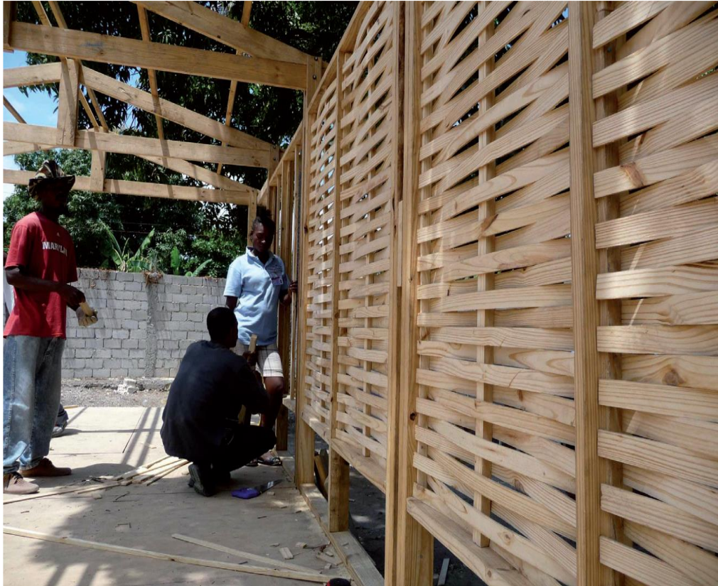
Figure 9.8 Source: (Sheltercasestudies, 2012, p. 33). The local workers used the traditional model referred to as ‘classide’, in building the shelters.
