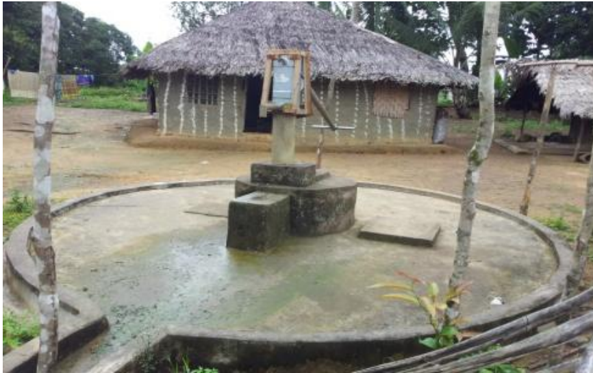
Hand Pump In District #4 Grabd Bassa County Constructed by the United Methodist Church picture taken August 7, 2012
